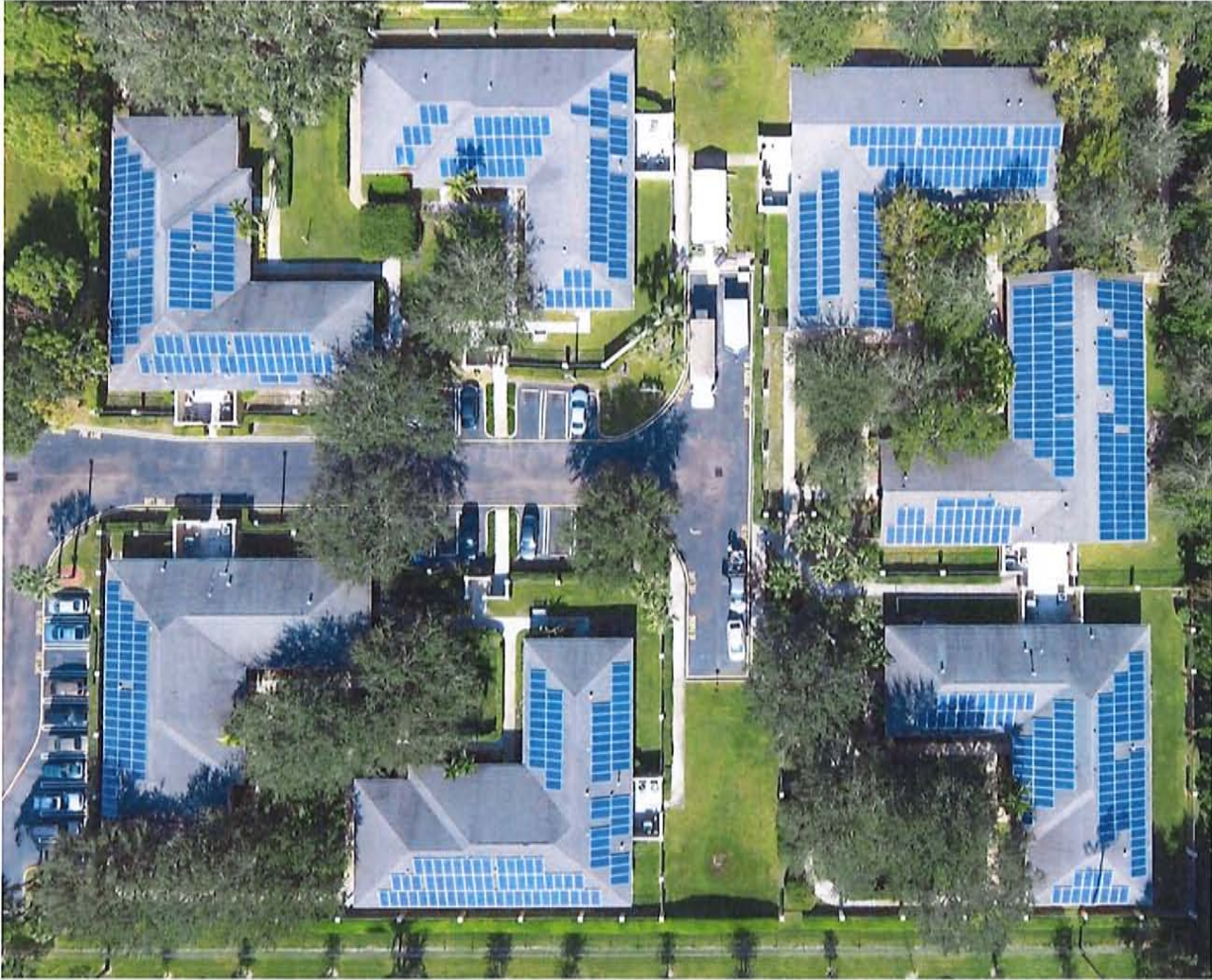
Pacifica Greenacres – 280kW flush mounted rooftop solar photovoltaic system
