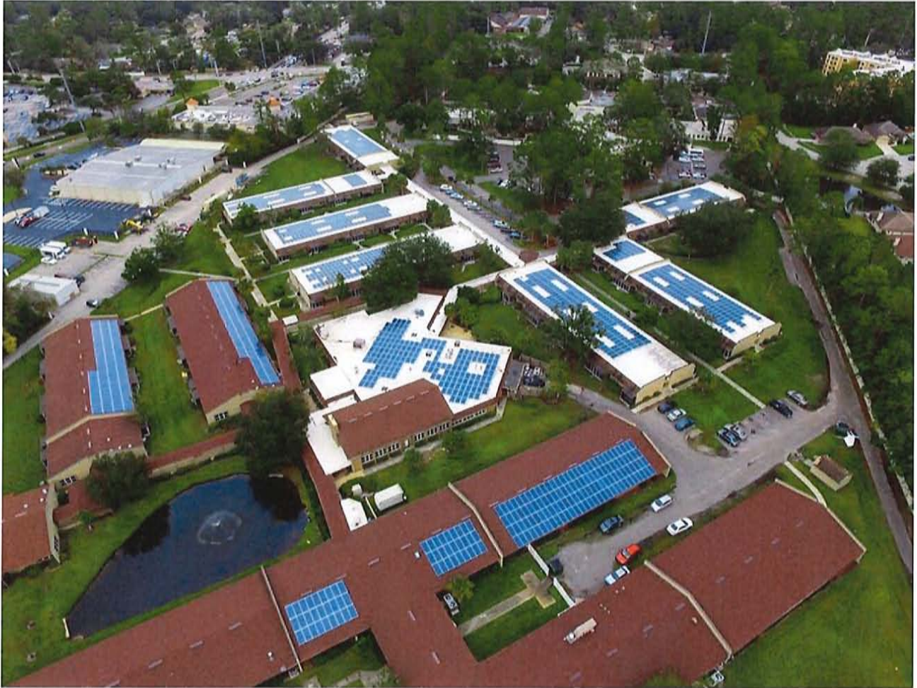
Pacifica Jacksonville – 570kW rooftop ballast and flush mounted solar photovoltaic system
