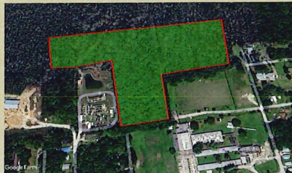
Hastings Water Treatment
